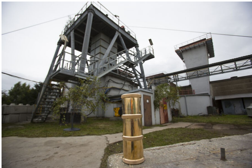
Figure: A photo of the ventillation shaft [4]
